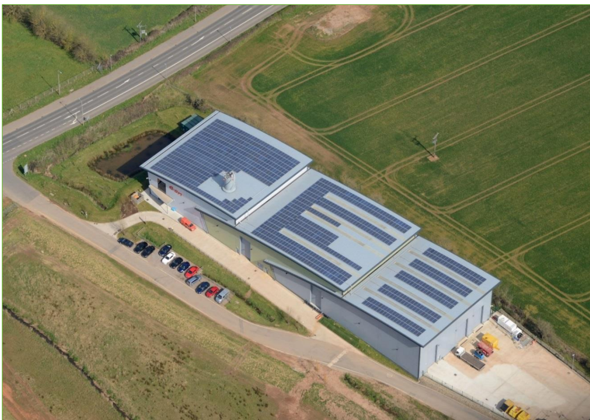
Figure 5 - Aerial photograph of the existing Energy Centre which serves Cranbrook on a district heating network. The land to the right of the energy centre is the western extent of the Treasbeare Expansion Area. (Image credit: Still Imaging)
