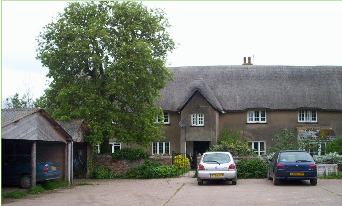
Figure 14 – Grade II listed Tillhouse Farmhouse, located in phase 2 of Cranbrook, south of the Country Park
